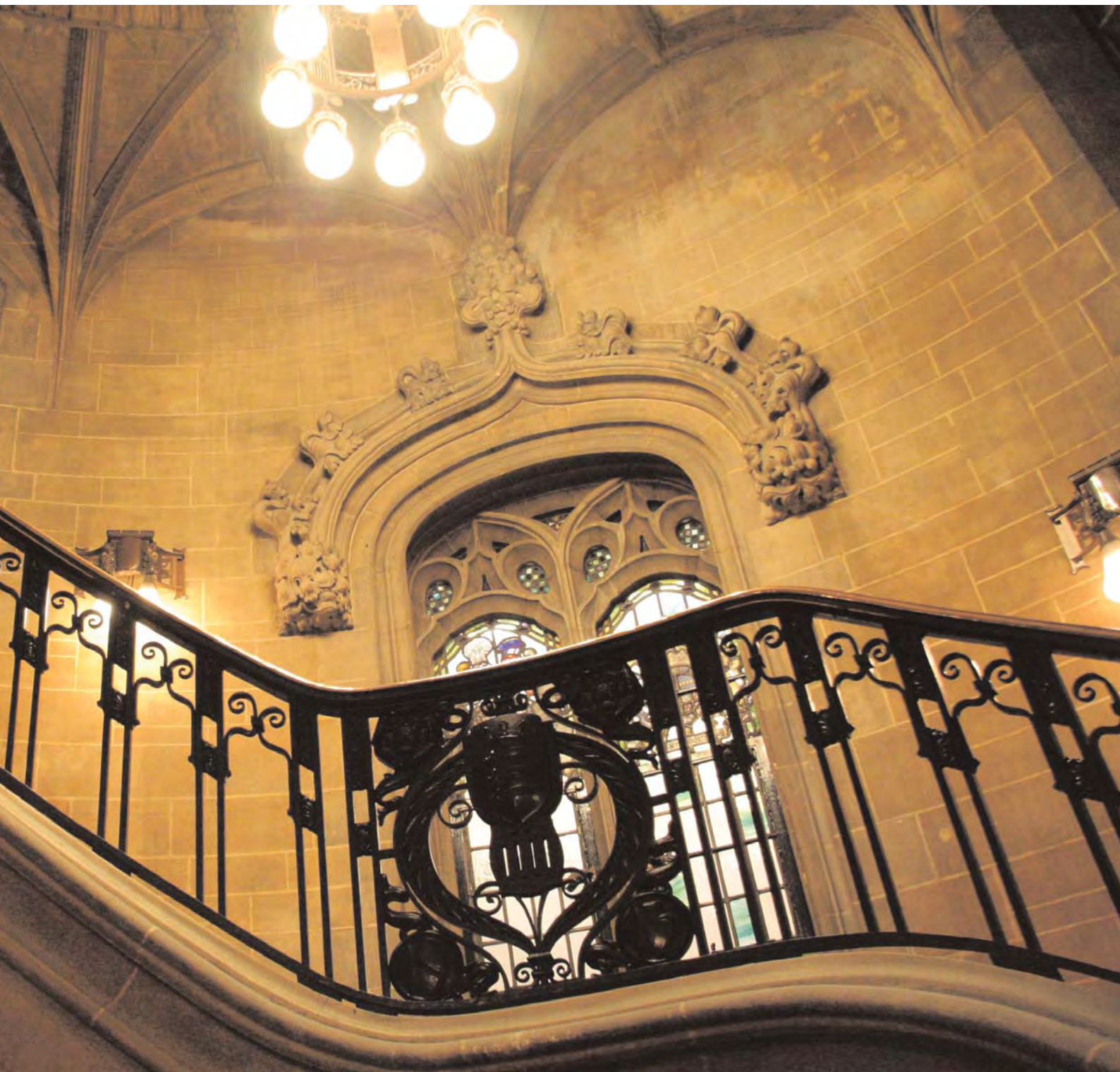
The main staircase illustrates the quality of the ironwork, fittings and fixtures. The walls are stucco imitating stone
