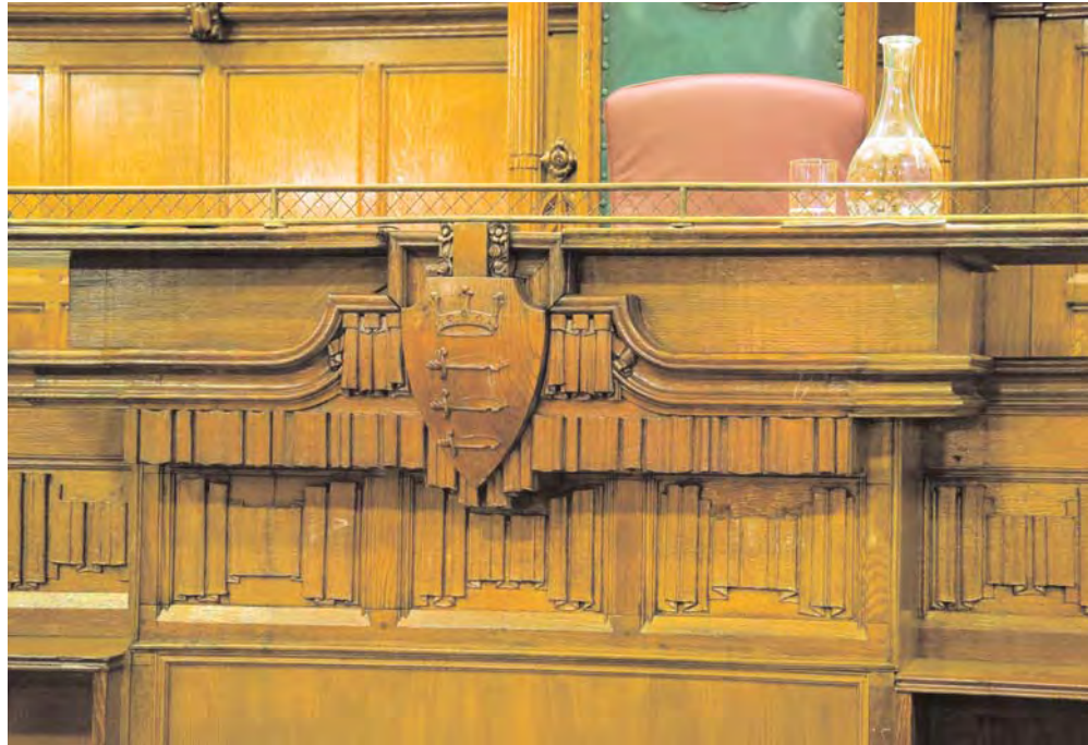
The intricately carved linenfold panelling and Middlesex coat of arms below the throne in Court 1
