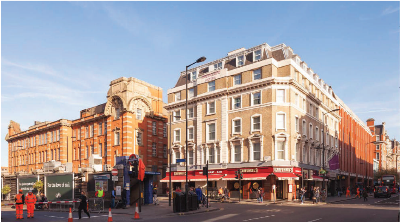
The existing Edwardian sorting office (left), a handsome building of merit in the conservation area
