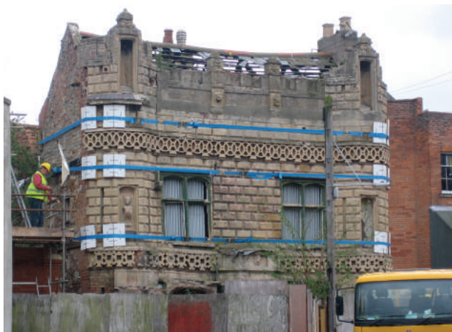
Works taking place at Castle House, Bridgwater
