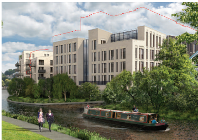
The revised proposal for the Newark Works. The red line indicates the size of the previous proposal.
