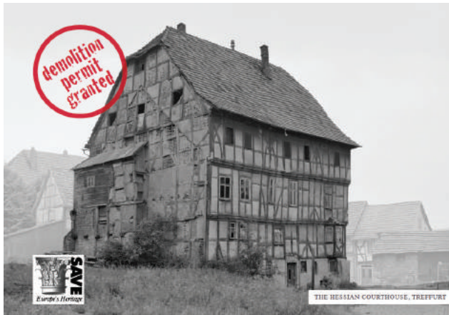
The cover of the SAVE Europe's Heritage report on the Hessian Courthouse
