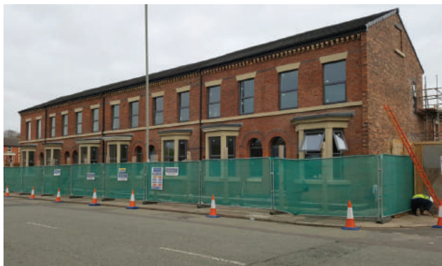
The pilot scheme on High Park Street nearing completion.
